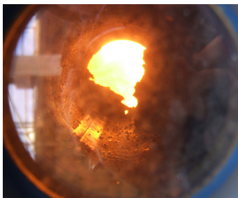
Wood is burned in the boiler to generate steam.
